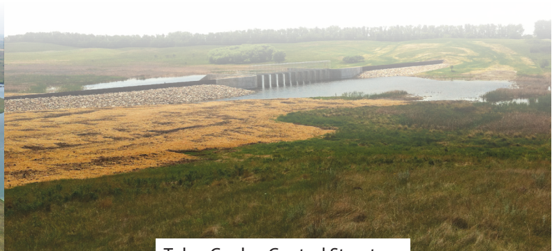
Tolna Coulee Control Structure
